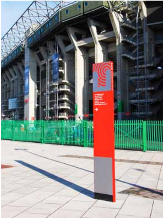
In 2009 Rivermeade successfully completed the resigning of Twickenham Stadium and the adjoining Marriott Hotel.
